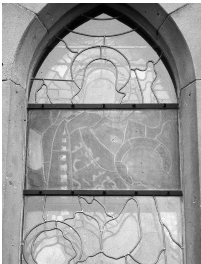
Exterior view of window with aesthetic glazing in central panel, New Kilpatrick Church, Bearsden, Glasgow. Photo: Mark Bambrough
